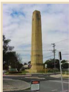
Lincoln Street Ventilating Tower
