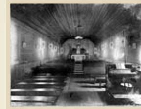
Interior of original Sacred Heart Church Mary Street, Highgate
